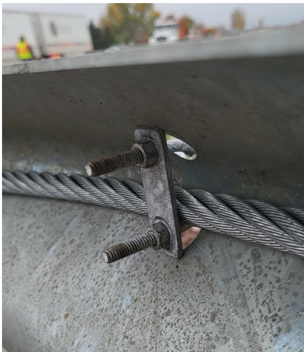
Figure 46. Nose Cable U-bolt Orientation
