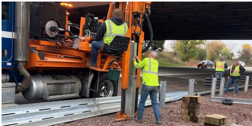
Figure 49. Driving UBSPs
