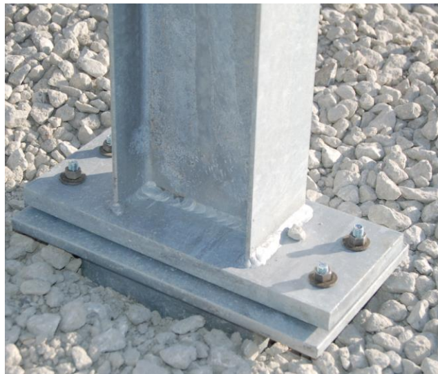
Figure 10. Assembled (top) and Installed (middle, bottom) UBSPs
