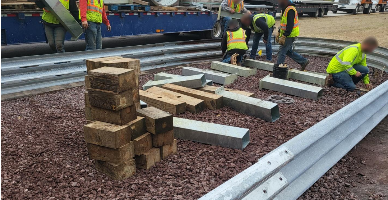
Figure 40. Posts and Blockouts in Approximate Final Location
