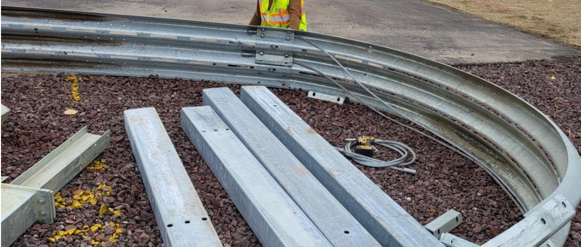
Figure 45. Partial Nose Cable Installation
