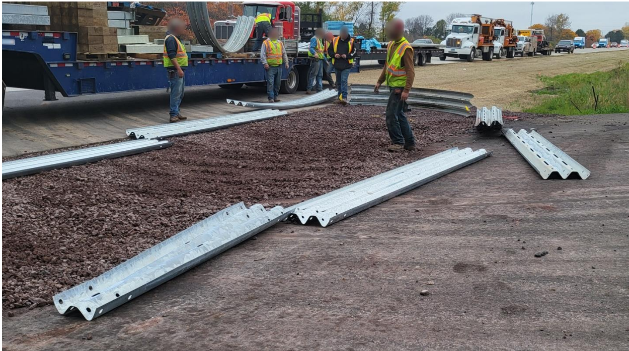
Figure 39. Guardrail in Approximate Final Location
