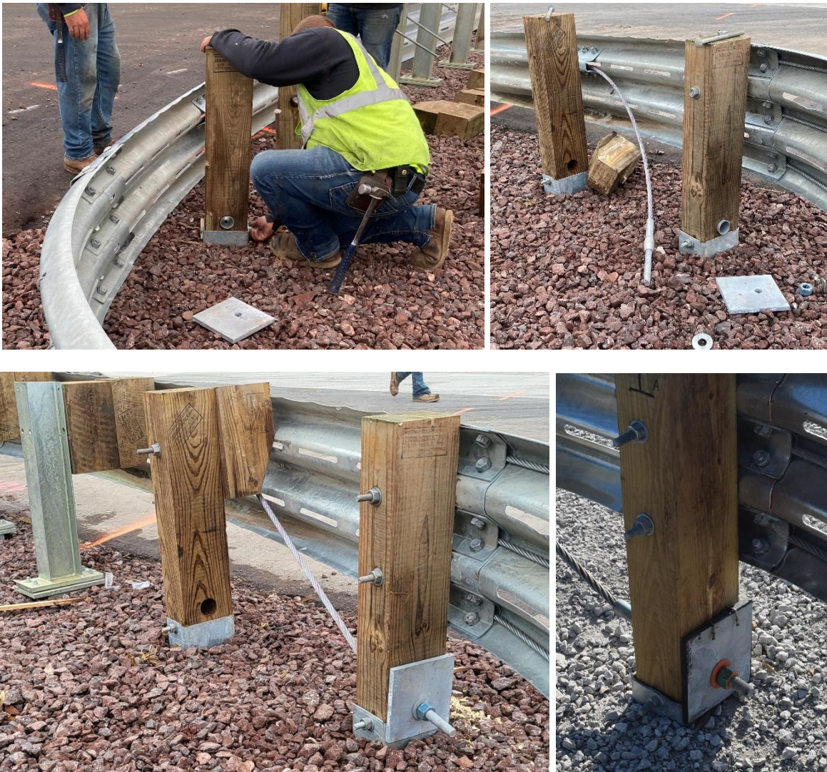
Figure 52. Cable Anchorage Installation
