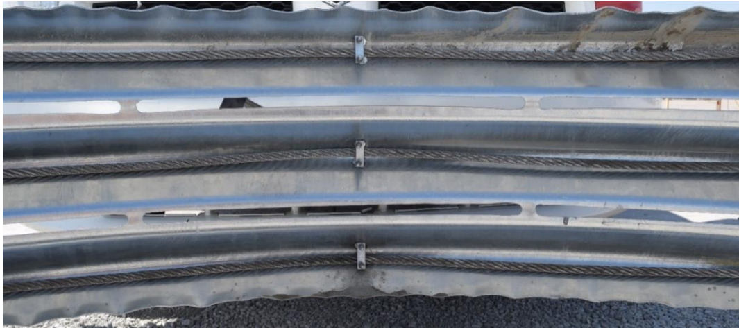
Figure 28. Cables Lining System Nose (Back View)
