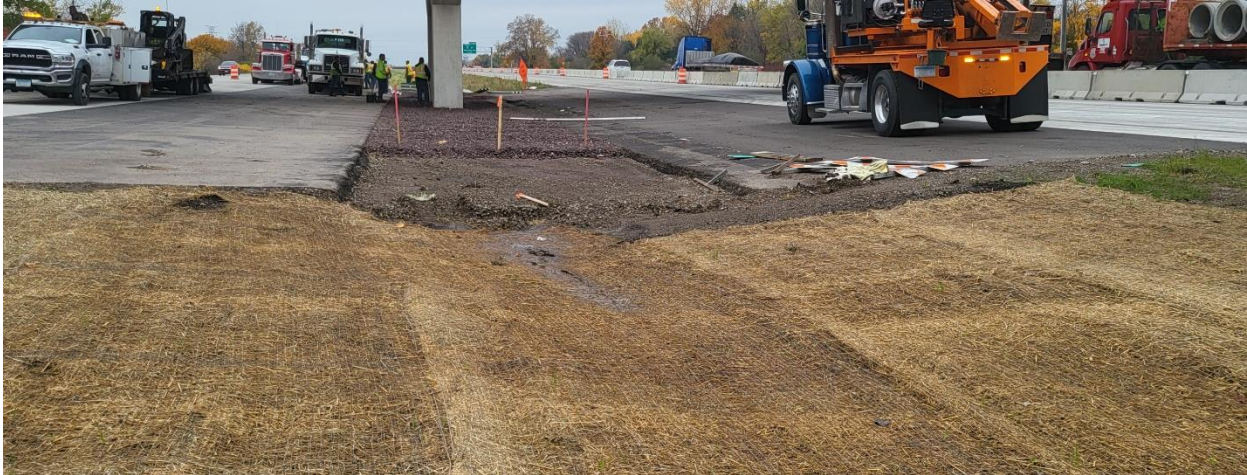
Figure 38. Site Grading with Nose Location Staked Out
