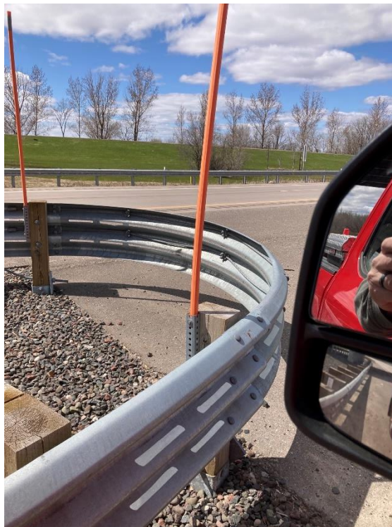
Figure 53. Snow Marker Installation
