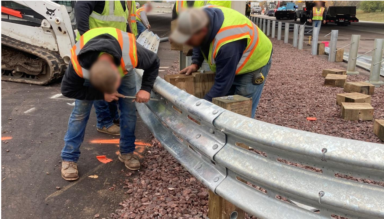
Figure 51. Attaching Blockouts and Installing Guardrail
