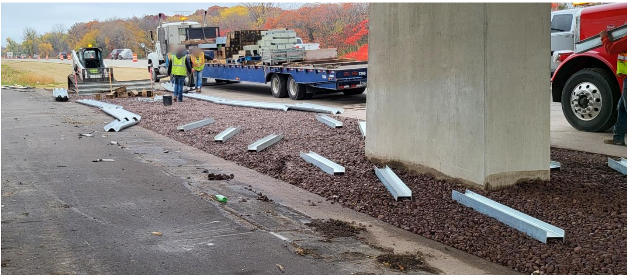
Figure 41. Posts in Approximate Final Location
