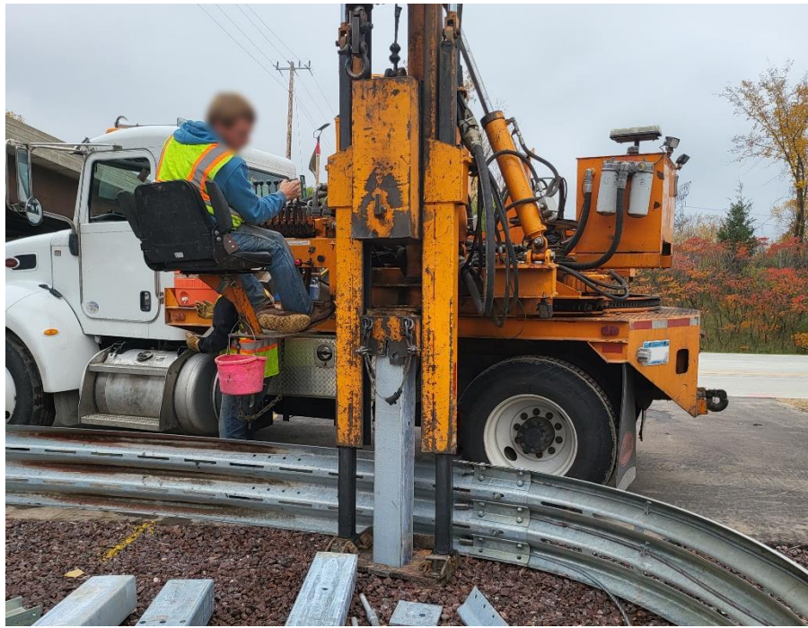
Figure 47. Driving BCT Foundation Tubes
