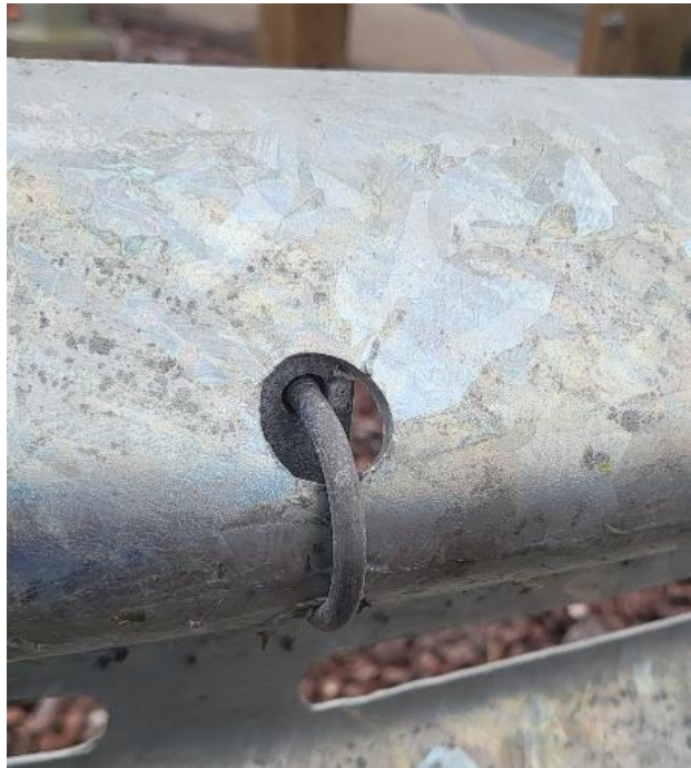
Figure 46. Nose Cable U-bolt Orientation
