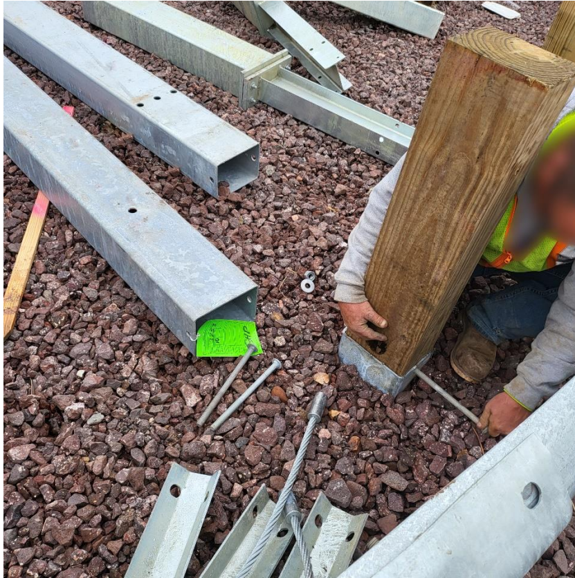
Figure 48. Installation of BCT Post in Foundation Tube
